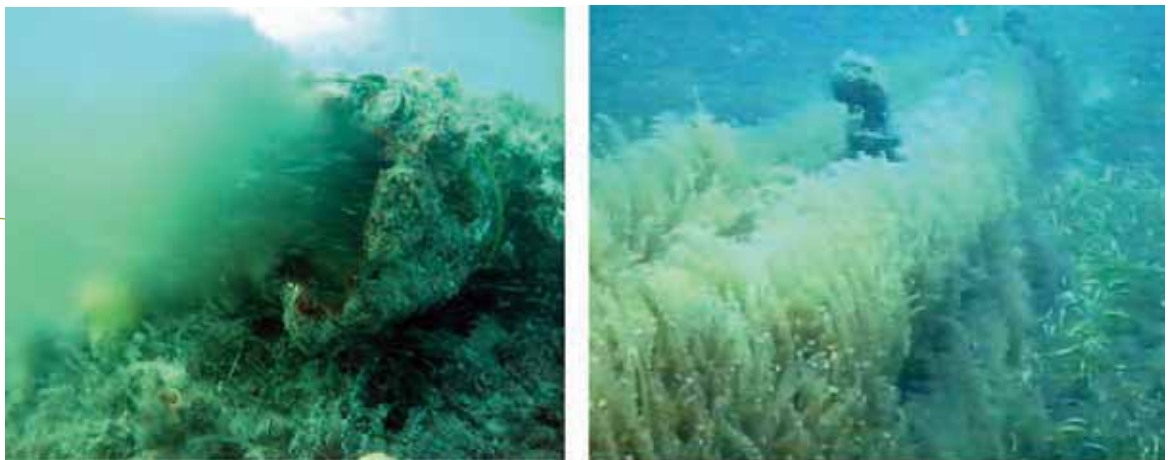
Figure 2: Examples of diffusers: Swanbourne outlet (left), which has been in place for decades, and is heavily covered in marine growth. Bunbury outlet (right) shown within 6 months of construction in 2001, the outlet is now also extensively covered in marine growth. Outlet pipes function as artificial reef structures, attracting fish and crustaceans.
